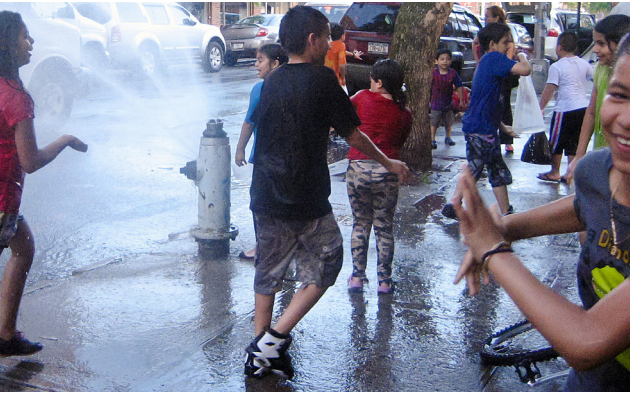
Fire hydrants throughout community
