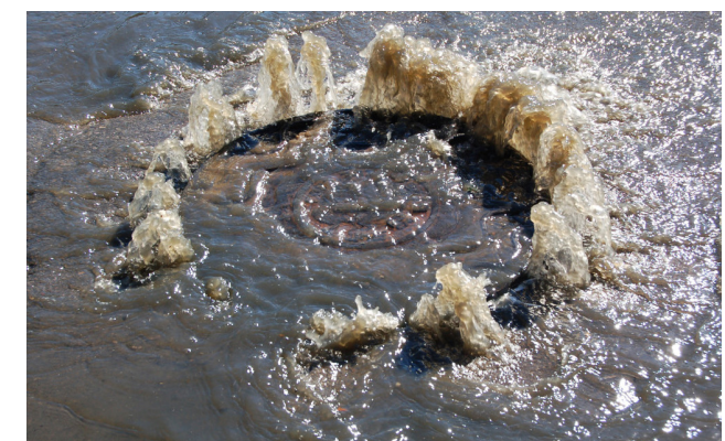
Street-level sewage backup
